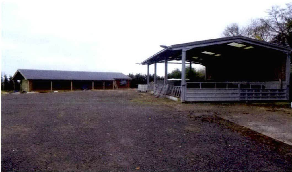
Existing lairage building with log cabin in the background
